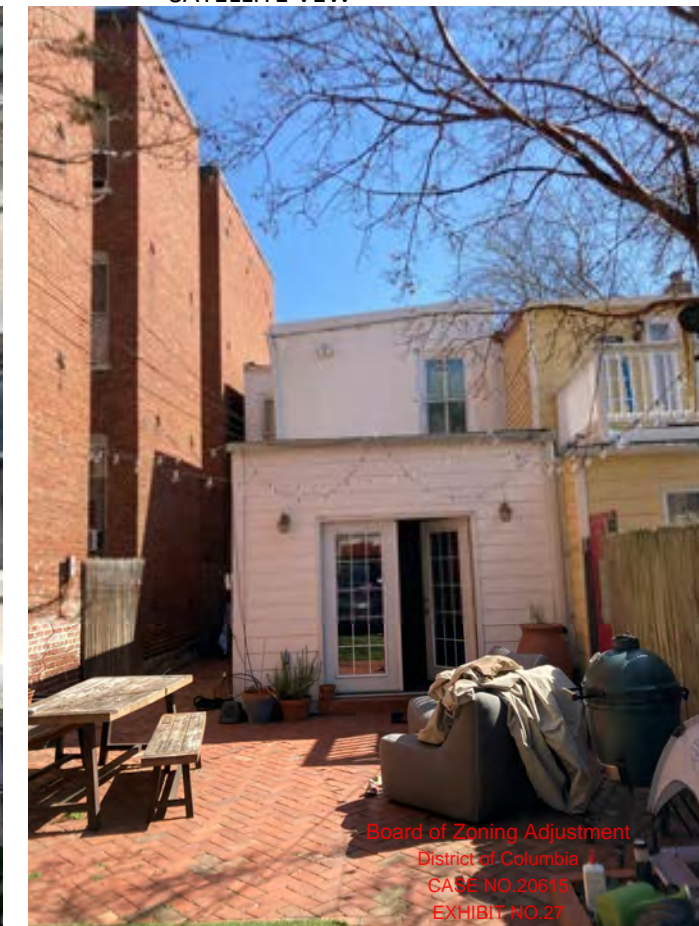
EXISTING REAR FACADE
