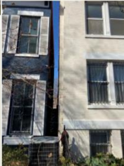
WALKWAY BETWEEN 751 AND 747
