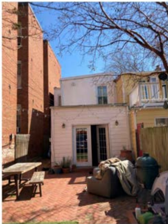
EXISTING REAR FACADE
