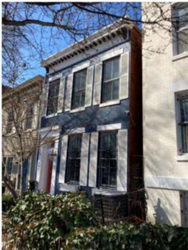
EXISTING FRONT FACADE
