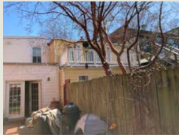
REAR FAÇADE, LOOKING SOUTH
