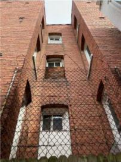
LIGHT WELL AT 747 10 TH SE
